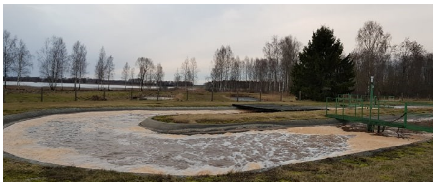
AS Linda Nektari reoveepuhasti ringkanal
